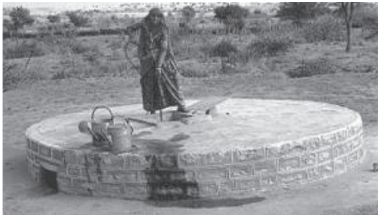
Tanks with underground cistern
