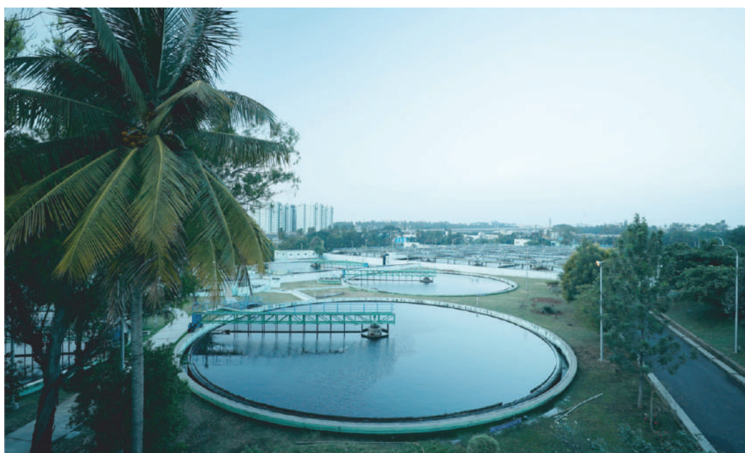
Fig. 20.8. Sewage water treatment plant
