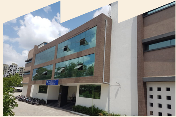
Regional Office & COE Pune RLM Business Park, SR.NO. 28/ 4/A, Old Kharadi Mundava Road, Kharadi, Pune, Maharashtra - 411014
