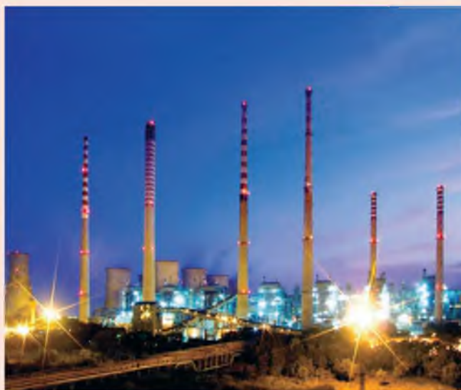
Raichur Thermal Power Station
