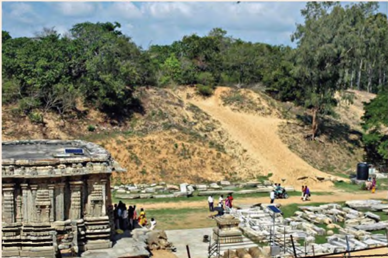
Renovation at Talakadu, T.N.Pura Taluk, Mysuru Dist.
