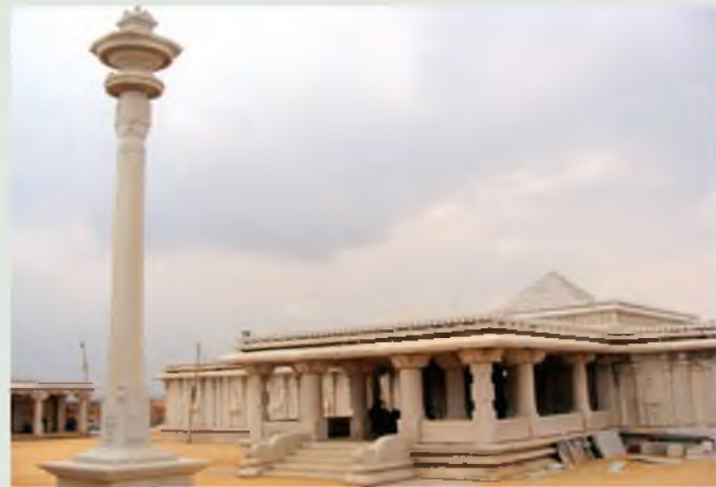
Gopalakrishna Temple After renovation, New Kannambadi
