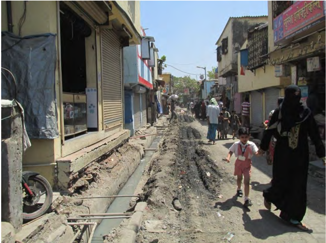
Filth, slush and muck with open drain used for defecation in the open at Govandi, Mumbai
