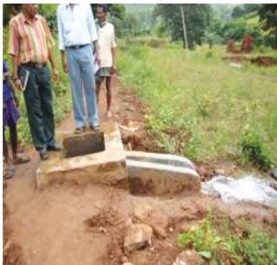
Outlet of a Diversion based irrigation project
