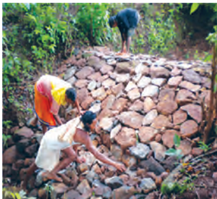
Loose Boulder Structure
