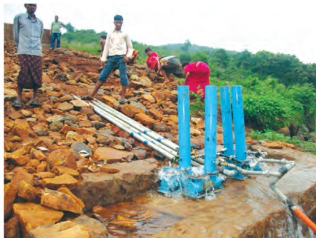
Operation of 4 nos. of hydrams in series
