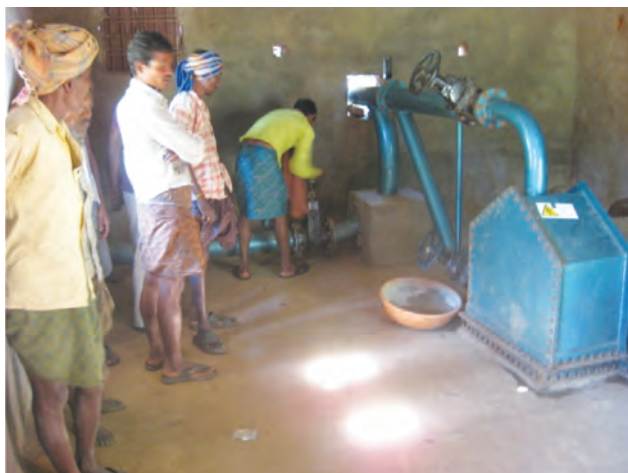
Micro hydro electricity project generating electricity
