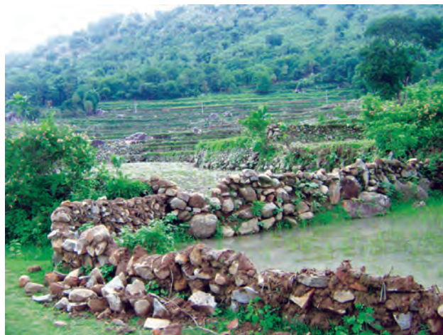
Land levelling with stone bunds
