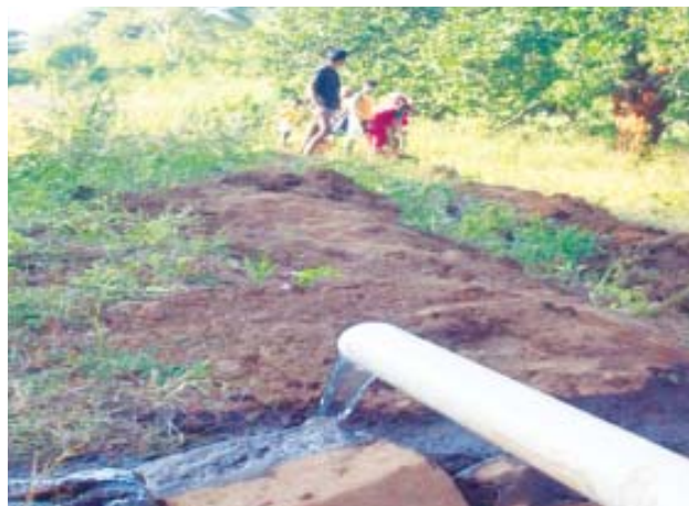
Ongoing burried pipe irrigation project
