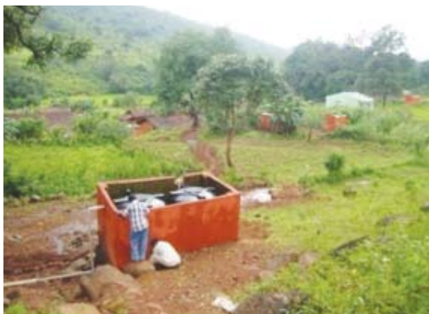
Gravity fed water supply system
