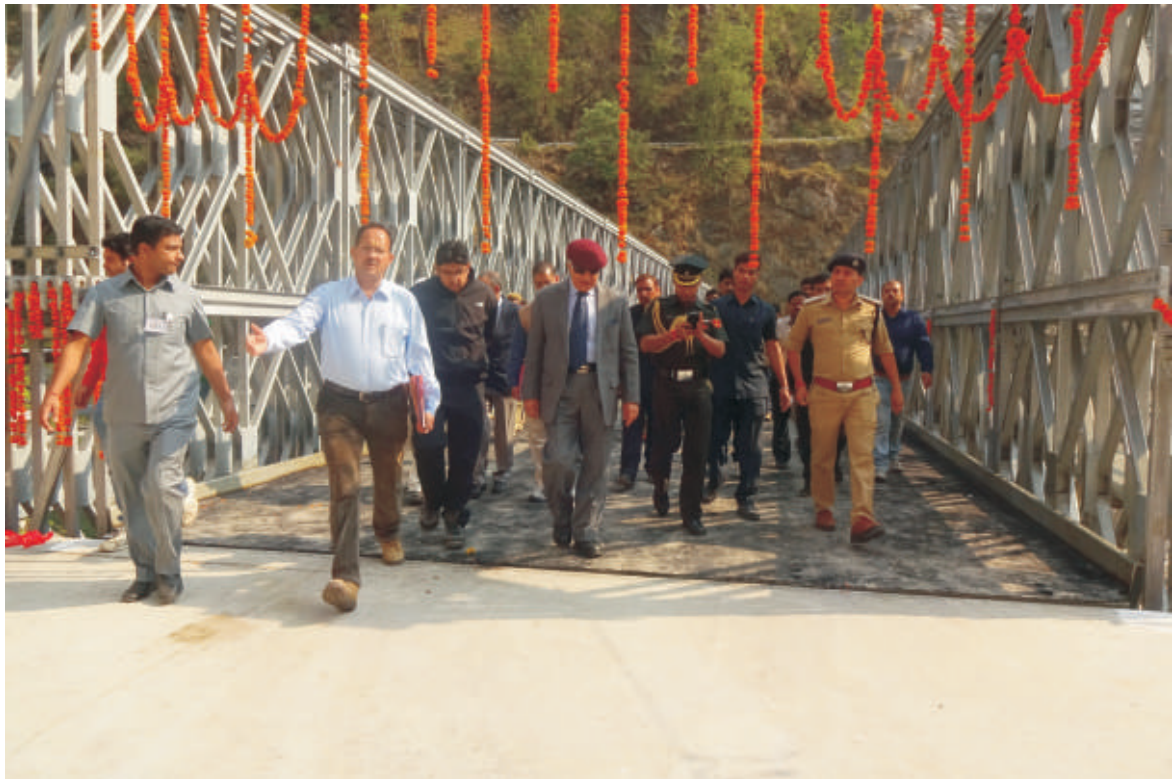
Inaugurating the newly built steel bridge on the Sonoganga at Soneprayag on the Kedarnath Dham route - 9 May 2016
