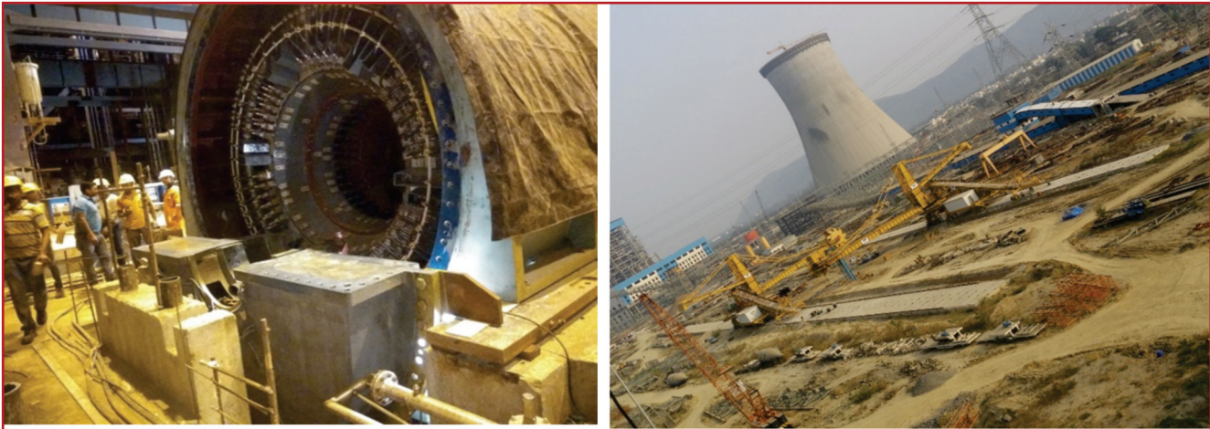
Works at Kothagudem Thermal Power Station – VII (1X800 MW )
