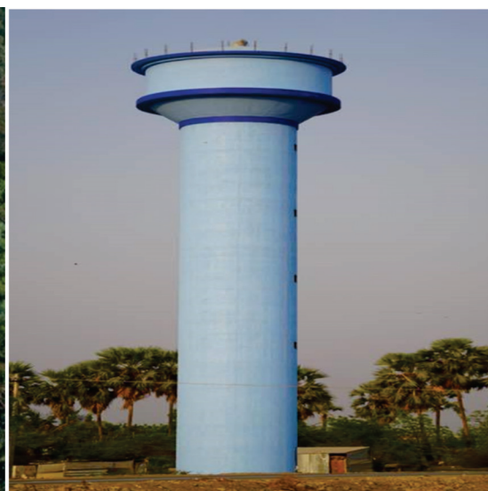
200 KL OHBR at Seetharampur Palair segment
