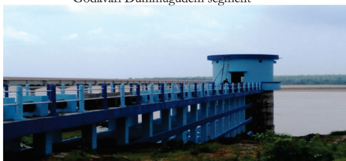
8-m-diameter Intake at Godavari Pusuru (Wazeedu Mandal) – Pusuru sub-segment – Khammam District
