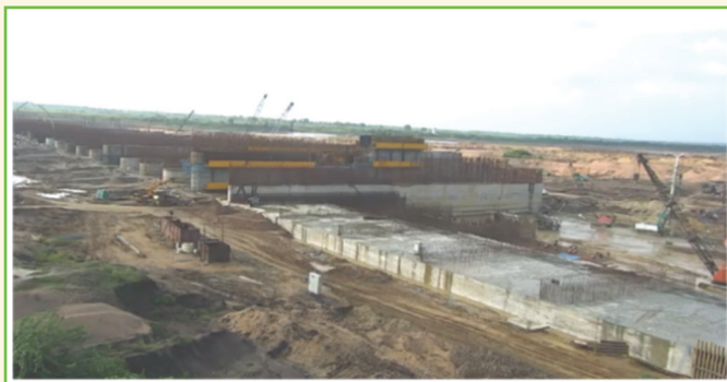
Annaram Barrage under construction
