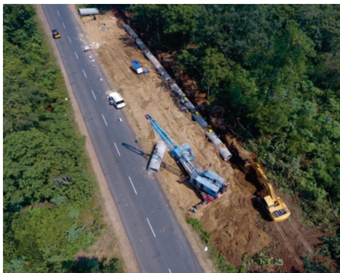
1500-mm-diameter PCCP pipeline Godavari Dummgudem segment
