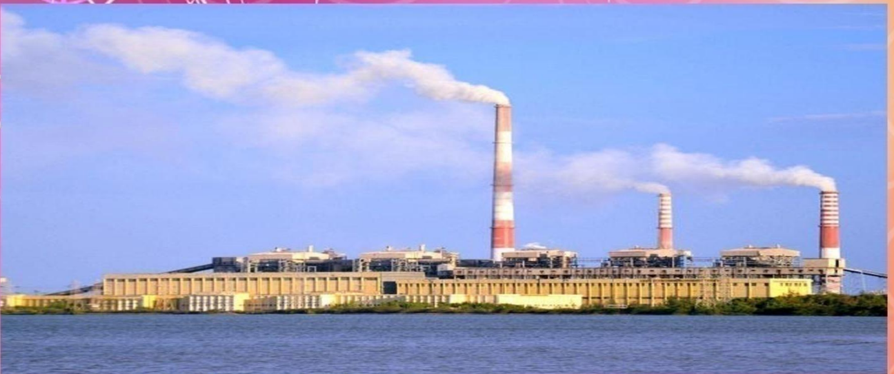
NTPL Power Station
