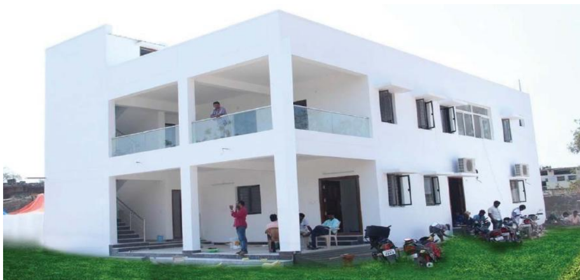
MLA Office- cum -Residence, Parkal
