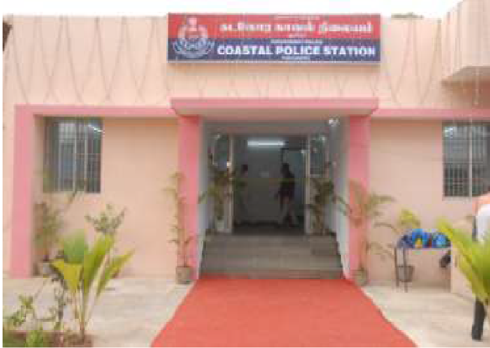
Coastal Police Station at Thengai Thittu Fishing Harbour, Puducherry
