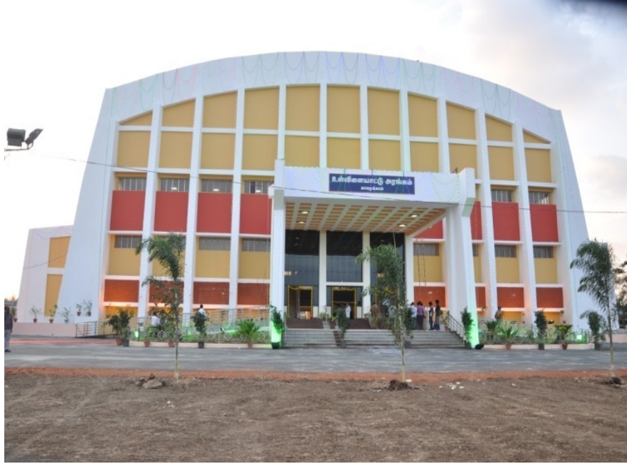
New Indoor Stadium at Keezhaveli, Karaikal
