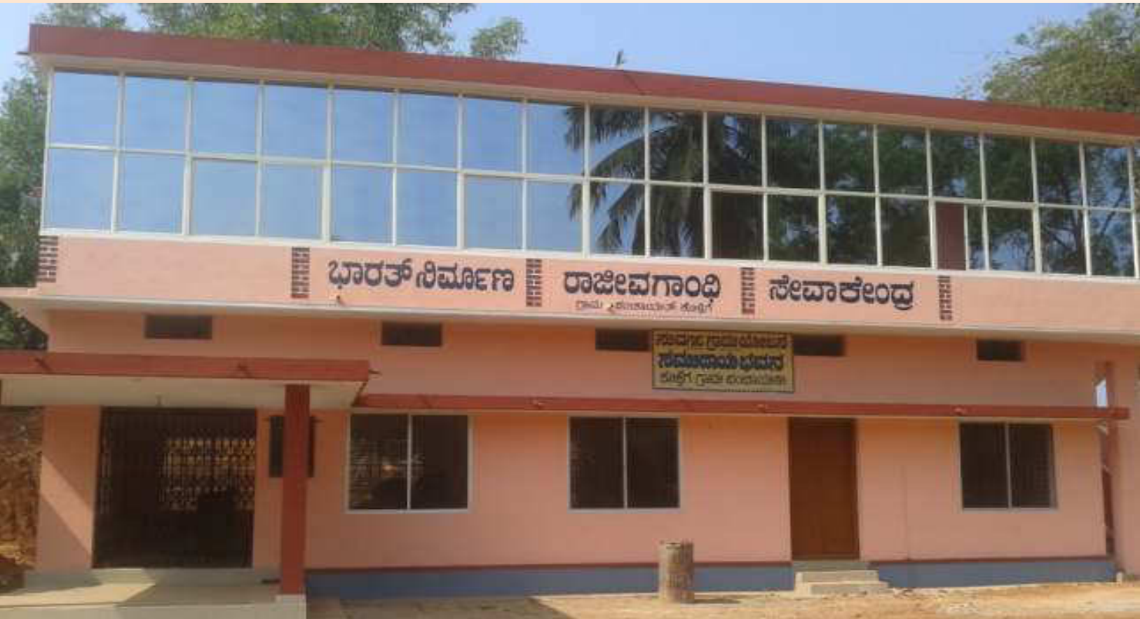
A Service centre and Rajiv Gandhi Seva Kendra at Kolthige Gram Panchayat - Puttur
