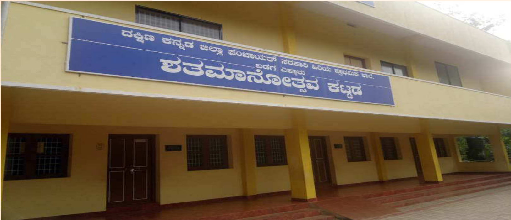
Govt. School Building
