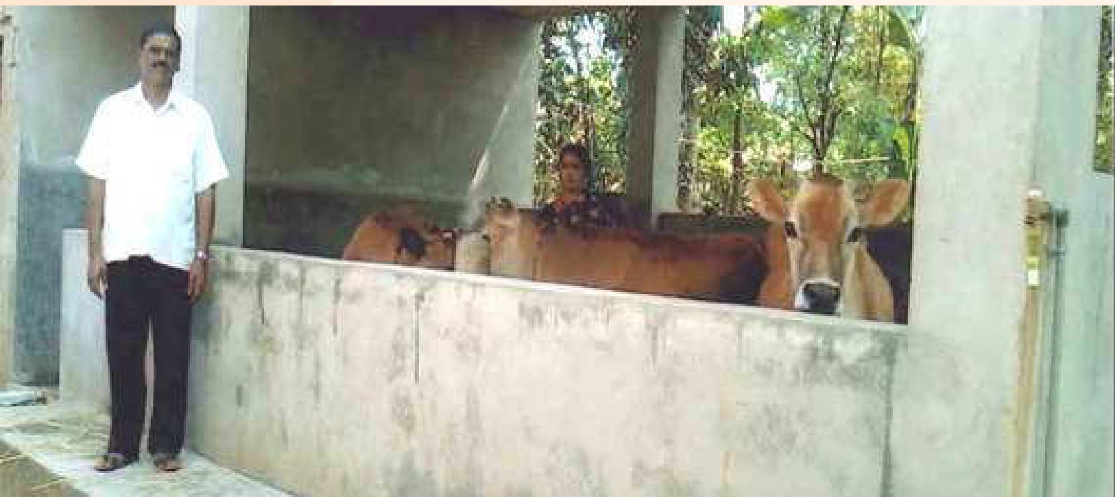
Cow Shed Construction Under MGNREGS
