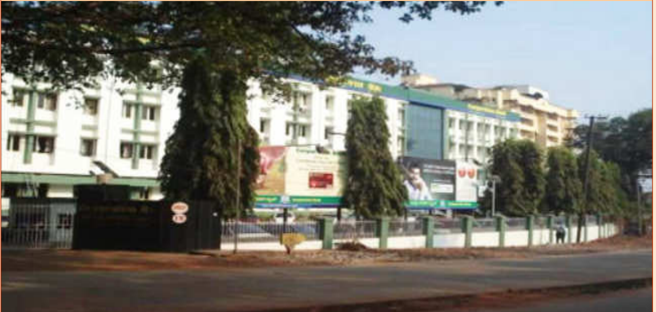
Corporation Bank Head office at Mangaluru
