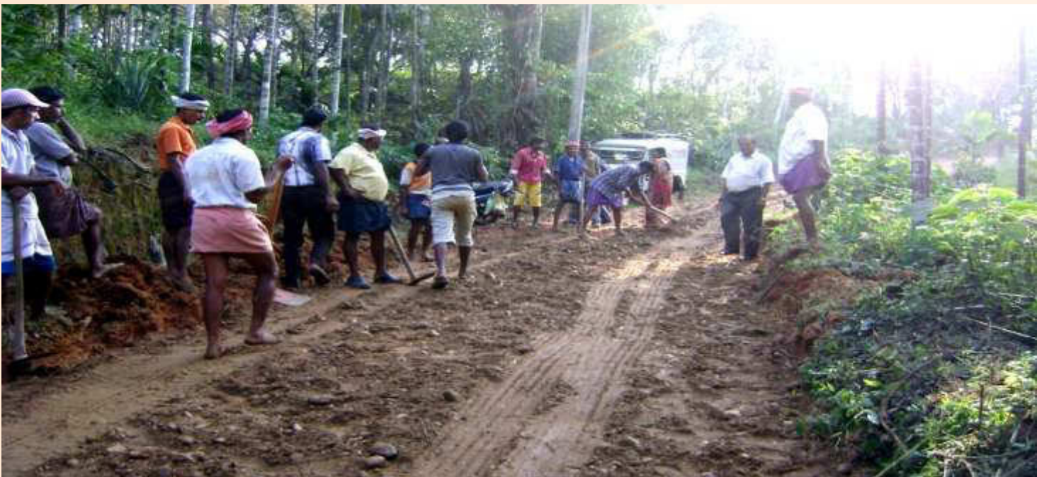
Road Construction Work under MGNREGS
