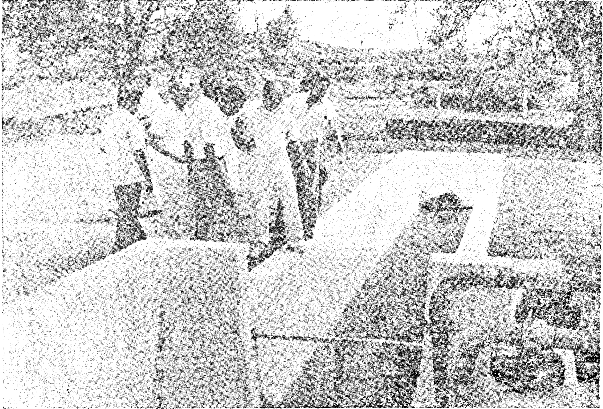
Madras Metropolitan water supply and Sewarage Board.
