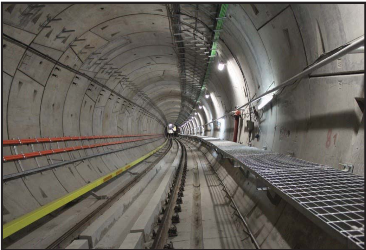
Tunnel of Metro
