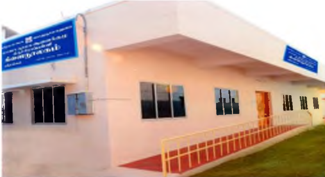
Picture 41. Branch Library, Srirangam, Thiruchirappalli District
