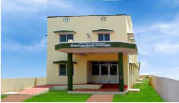
Picture 40 Branch Library, karaikudi, Sivagangai District
