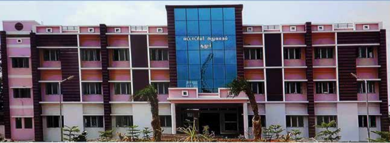
Taluk Office, Sular, Tirunelveli District
