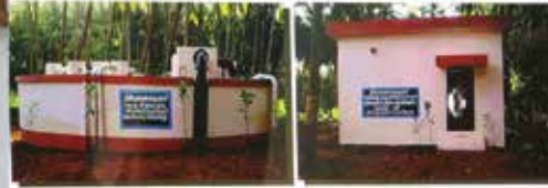
Dindigul Corporation - Aathur Additional Water Supply Scheme Ground Level Water Storage Tank and Electrical Motor Room
