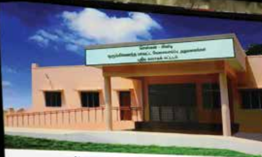
Chennai - Guindy Integrated District Employment Offices New Campus Building
