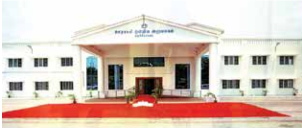
Panchayat Union Office Building, Pudukottai Union, Pudukottai District
