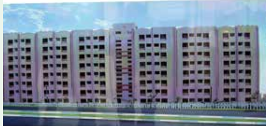
Tamil Nadu Slum Clearance Board New Multi-storeyed Building at Perumbakkam, Chennai
