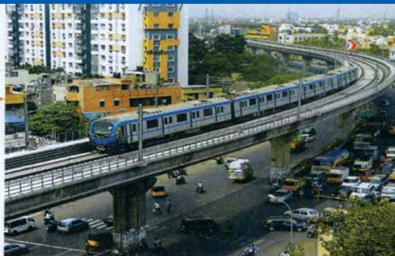
CHENNAI METRO RAIL DURING A TRIAL RUN
