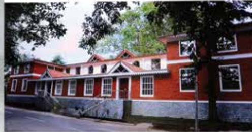
Kodaikanal Municipality - Office Building
