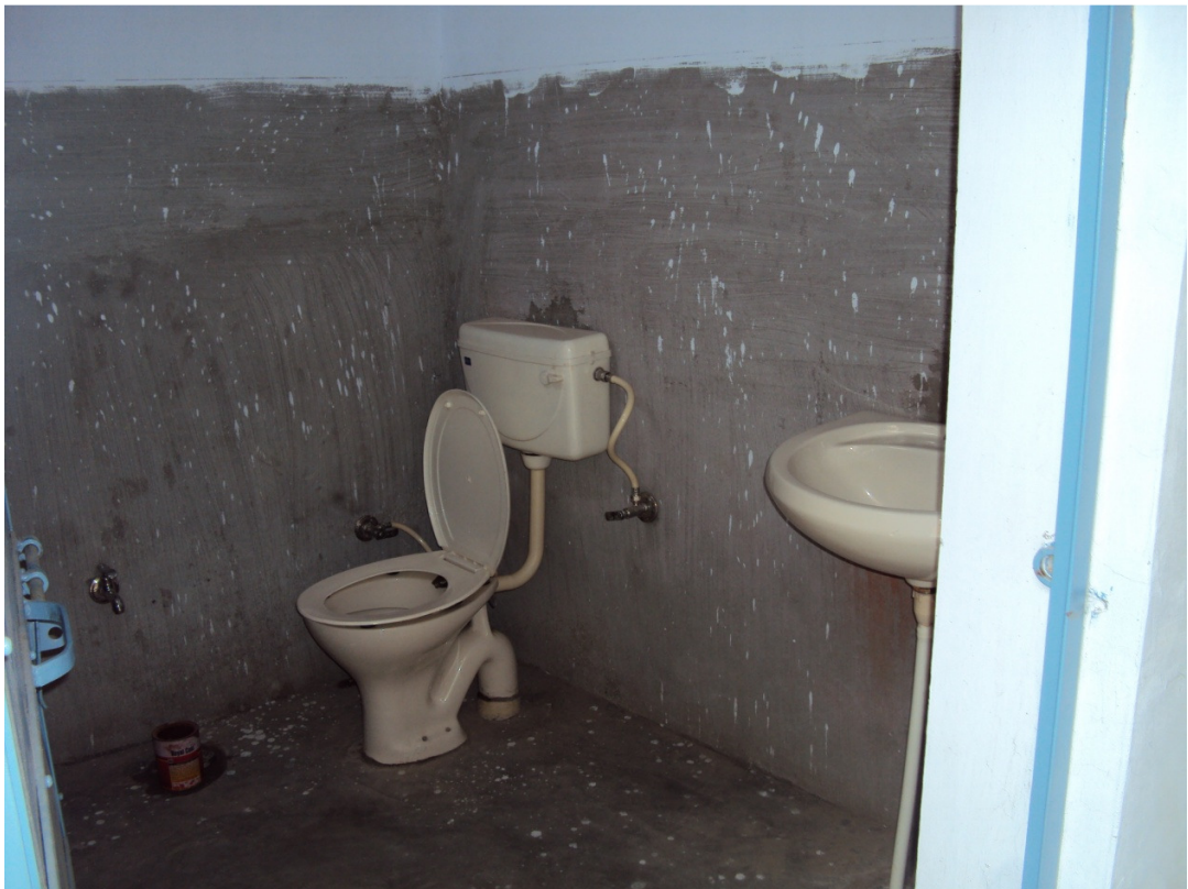
CWSN TOILETS WORK IN PROGRESS
