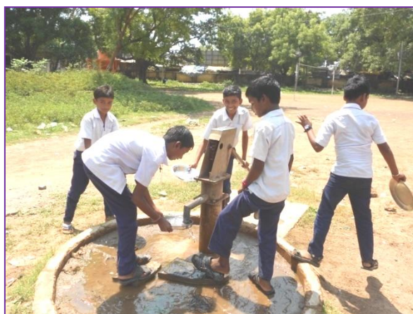
Water facility for Mid-Day-Meal at MS Kasdol
