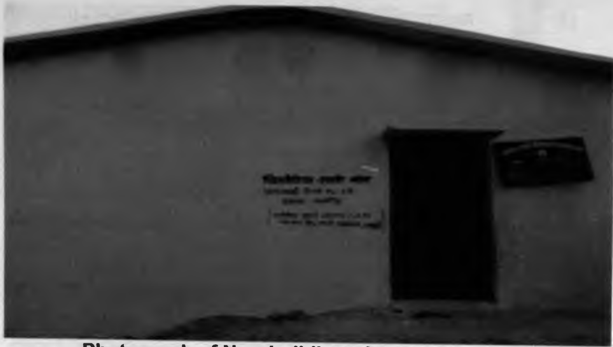
Photograph of New building of Aganbadi Centre (Picture No. 02)
