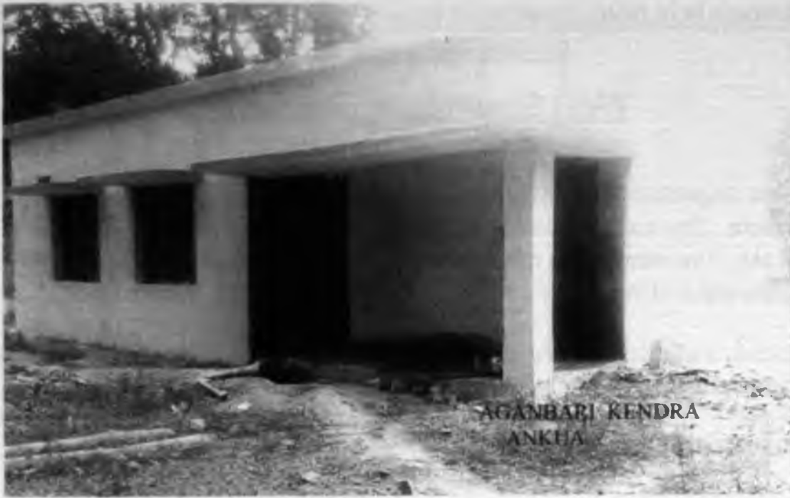
Aganwadi construction in Ankua village in chiriya panchayat in Manoharpur Block
