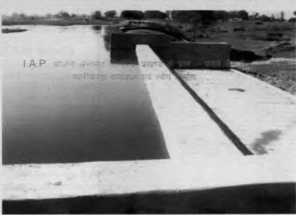
Pagar Dam After reconstruction
