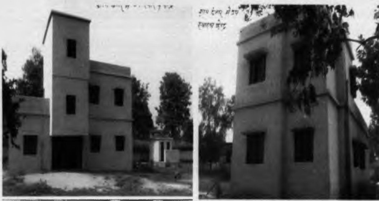
A typical HSC Constructed under IAP
