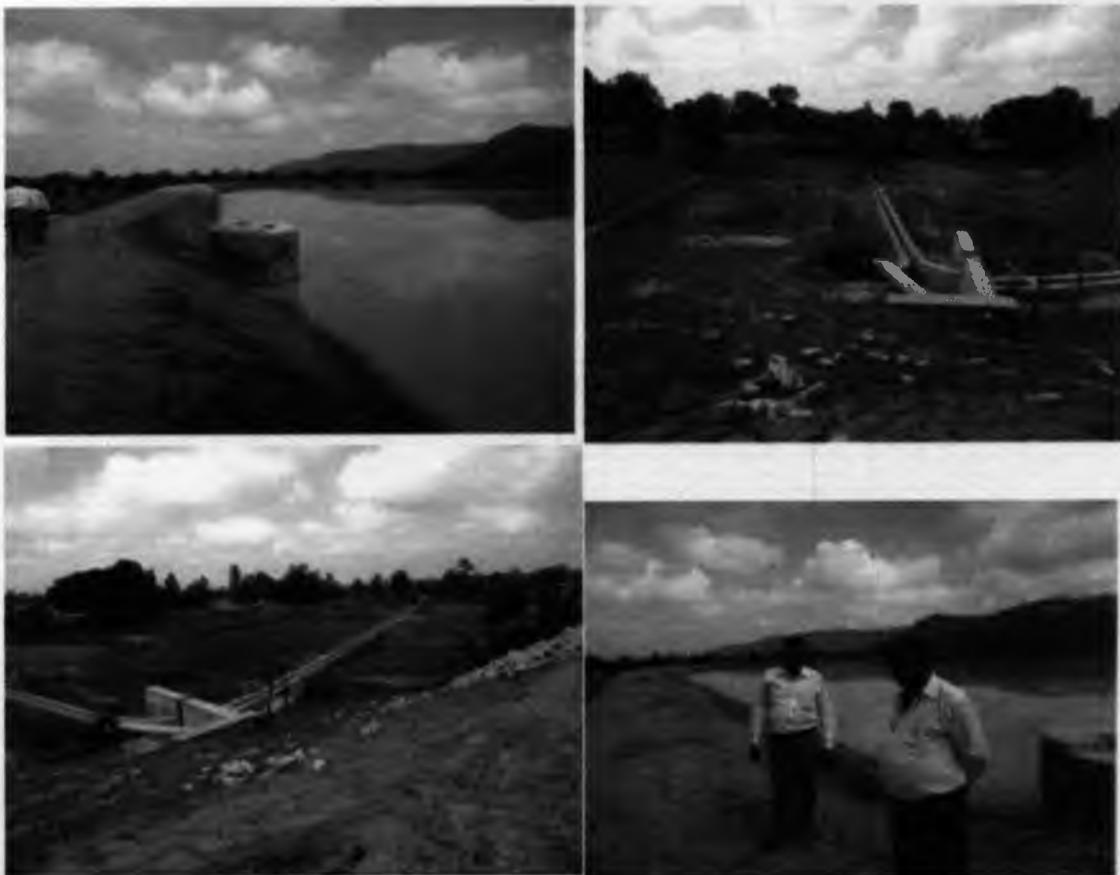
Photographs of Dam, Head regulator & Lined Canal.
