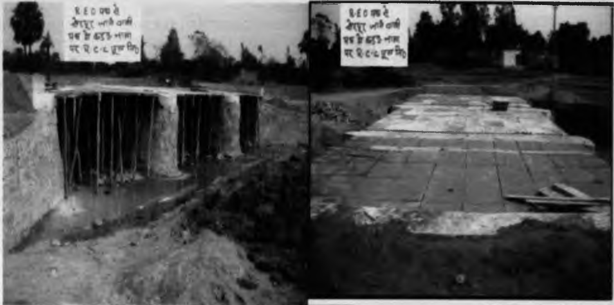
Construction of RCC Bridge near village Serpur on Kadrua Nala.
