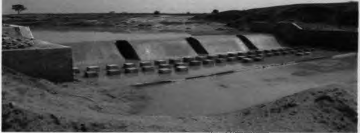
Bokta Nala Cheakdam Block - Bhandra Est. Cost - 23.405 Lakh
