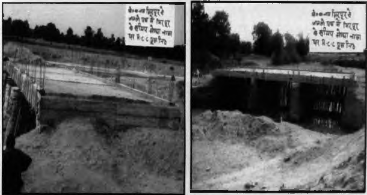
Construction of RCC Bridge near village Mirpur in Mirpur-Jajlo Road.
