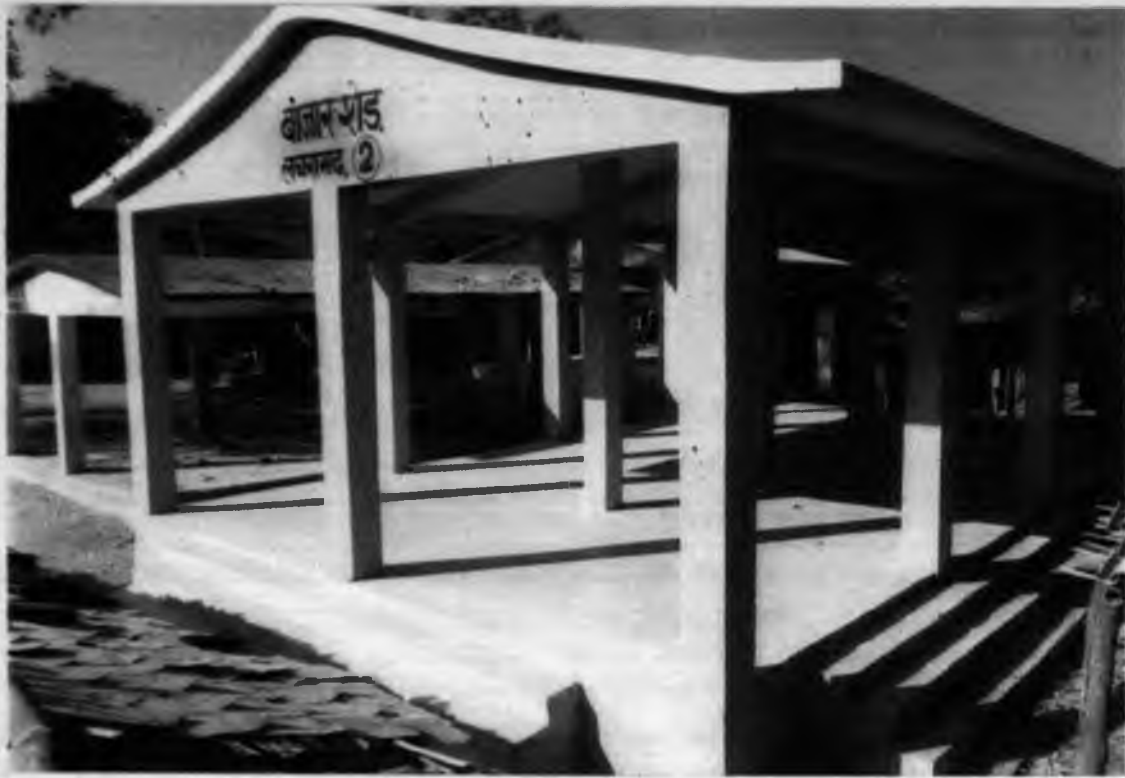
Photograph of Market Shed-at lachragarh
