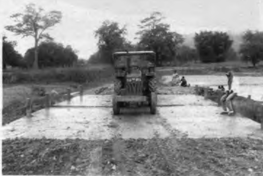
Goilkera –Orenga bridge, length – 2*15*8 ft RCC bridge in Goilkera Block
