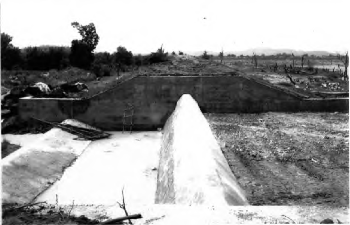
Talegaon MI Tank Waste Weir
