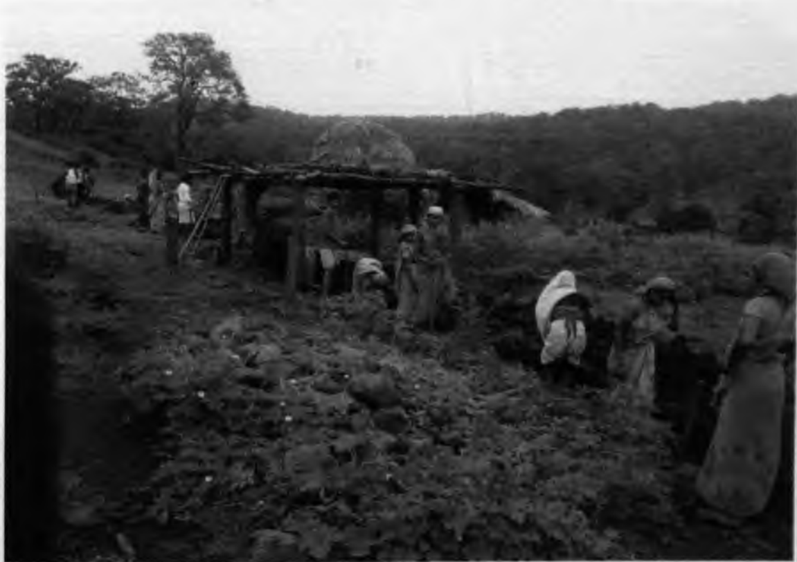
Digging of trench at Udhour
