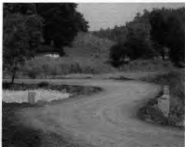
Road of Sunehra to Daldali (Rehtakhero State Border) Block- Mawai
