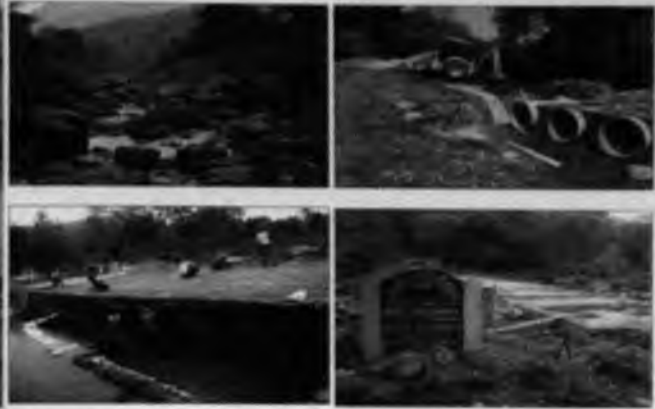
Construction of Vented Cause way on Baniabasa-Jenabil road
