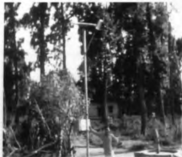
Establishment of Solar Street Lights - Sathiya village block Mawai
