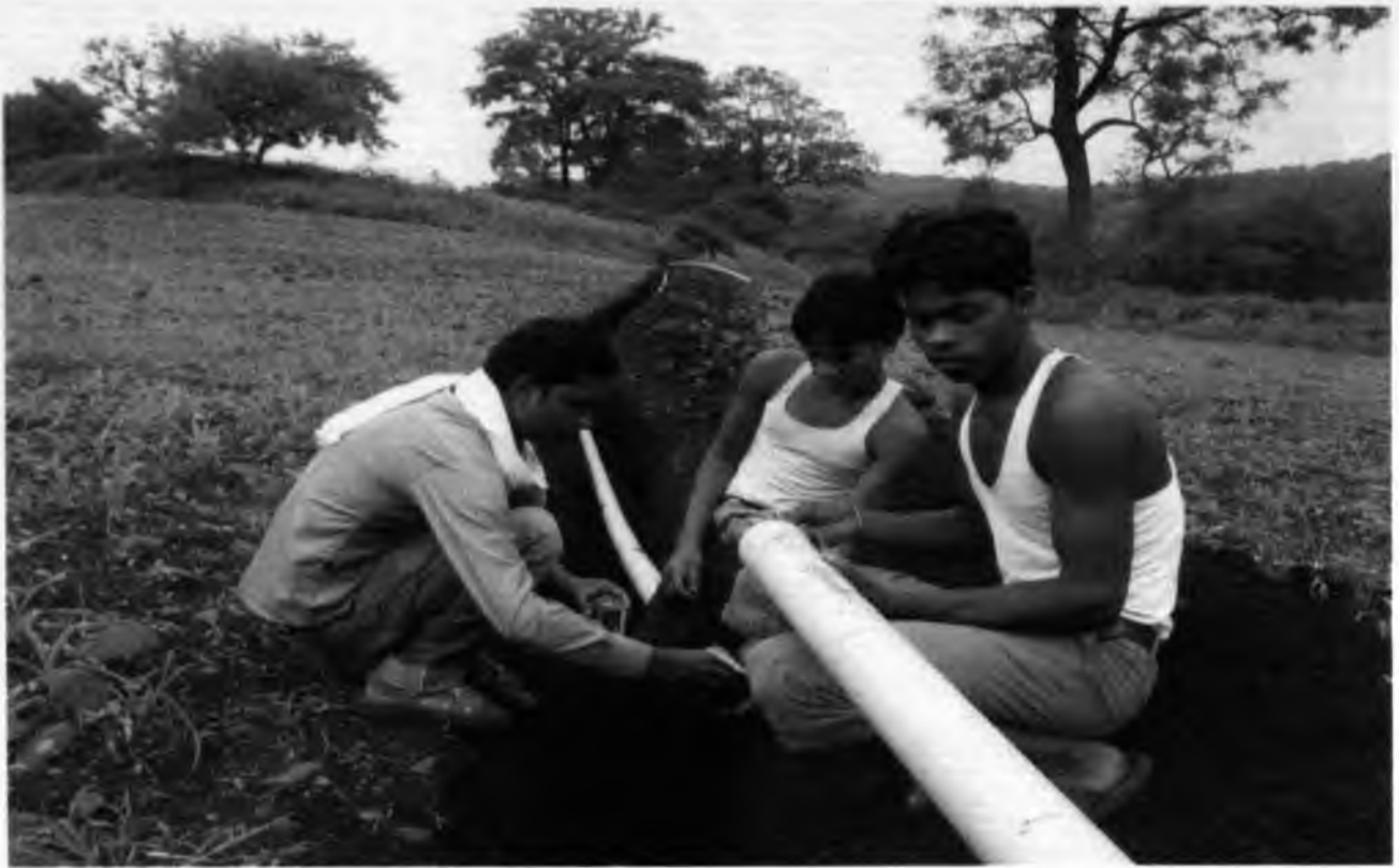
Fitting of pipes at Udhour
