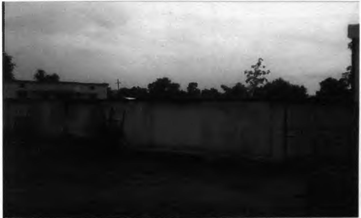
Wall Compound of ZP School at Mohali Tah: Dhanora
