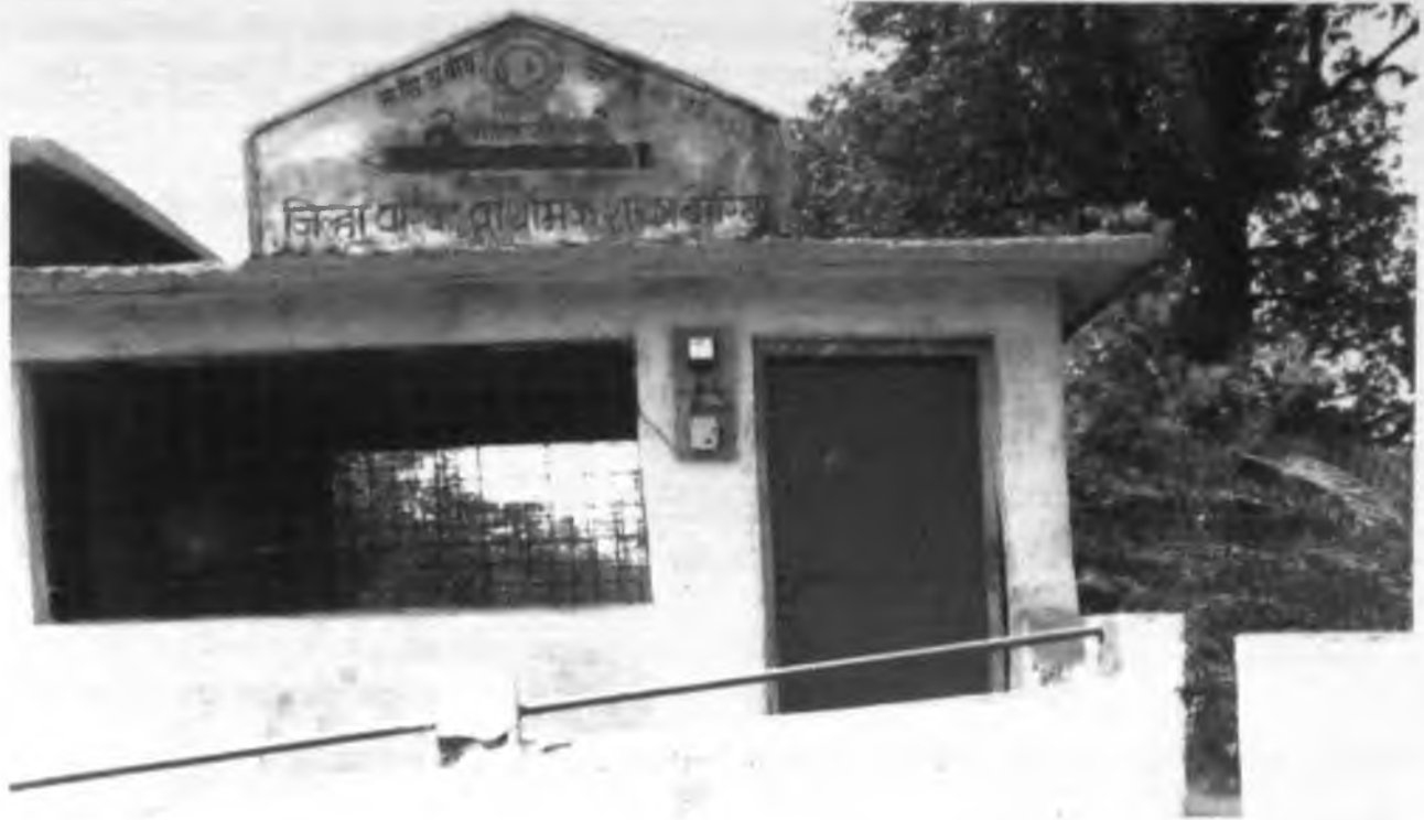
School Electrification- Z.P.Schooi, Boriya, Tah.Bhamaragad
