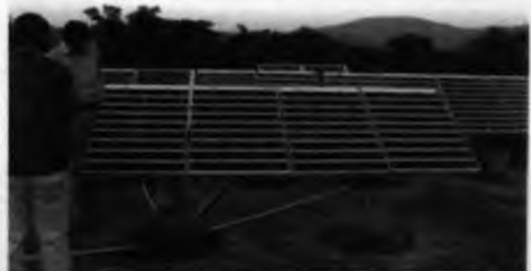
Solar panels installed in the ashram schools inside STR
