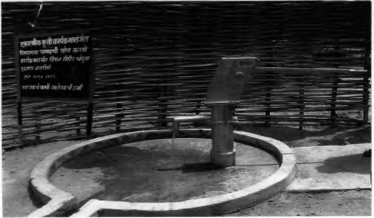
Drinking water Facility Z.P School, Dholdongari, Tah Korchi
