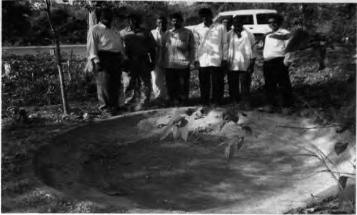
Construction of Water Pool at Nagalwahi Ta: Kurkheda
