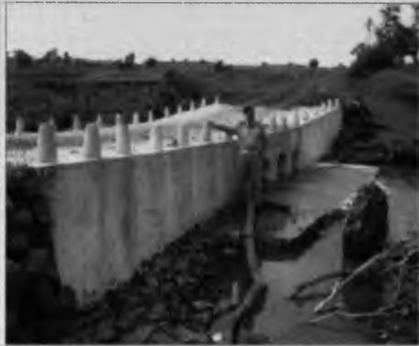
Culverts and bridges constructed inside STR
