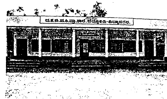
GLPS Bedrodi-Vidyanagar, Puttur Tq, Dakshina Kannada Dist
