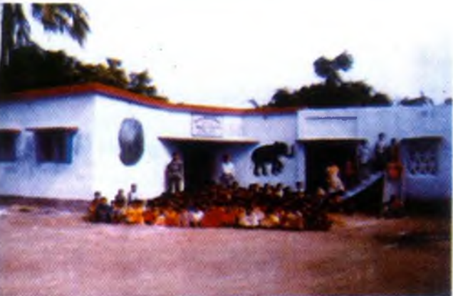
NEW SCHOOL BUILDING
