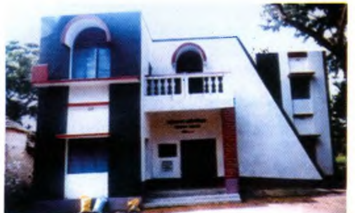
NEW SCHOOL BUILDING
